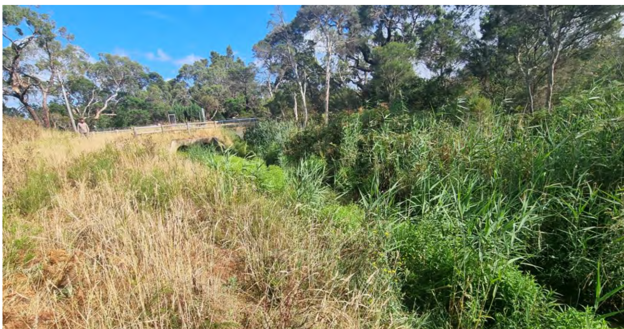
Photograph 3. Culvert beneath Tyabb-Tooradin Rd (photograph date: 12/2/2026)
